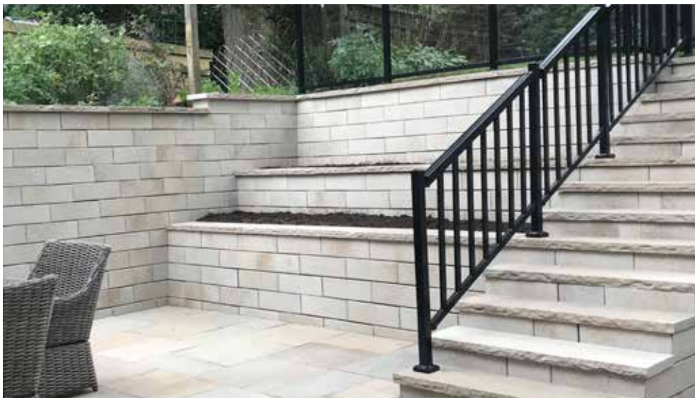
This sunken patio makes the most of its retaining wall with built in planters topped with Banas Flint coping. The Banas Flint patio in mixed sizes is a perfect complement to the manufactured stone walls surrounding it.
